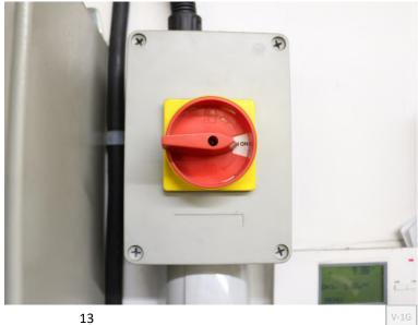
Turn **ON** the controller using the switch on the front panel. The controller will cycle through a start-up self-test during which the various indicators etc. on the front panel will flash, before settling to a display showing the last used setup.
