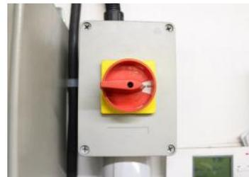
Turn **ON** the controller using the switch on the front panel. The controller will run through a start-up self-test during which the multi-function display will cycle through a welcome screen and show the current firmware version etc. also various indicators etc. on the front panel will flash, before settling to a display showing the last user setup. At this point the controller is ready to use at the settings employed during the previous operating period.
